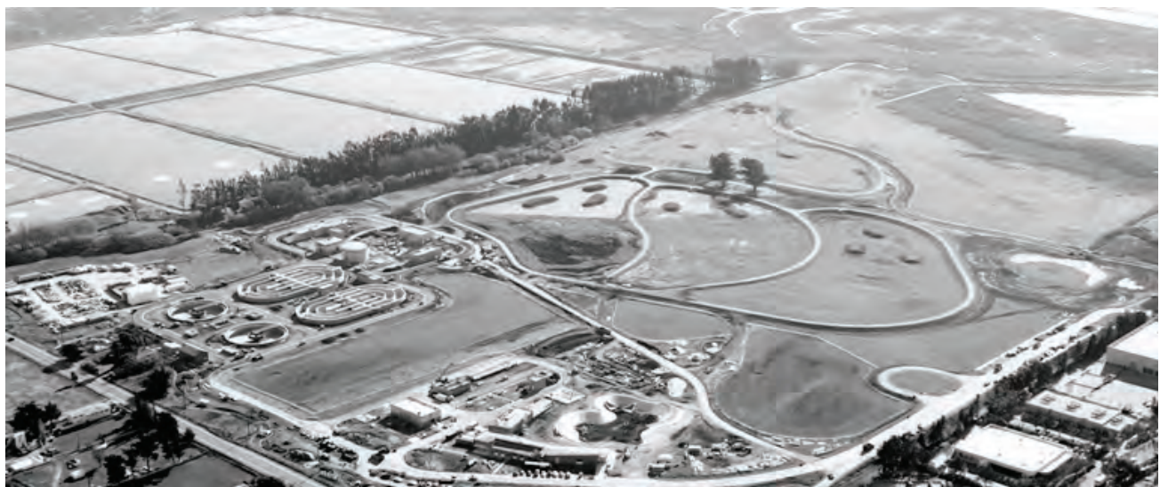
The Ellis Creek Water Recycling Facility, nearing completion, will provide tertiary recycled water to offset potable demand.
